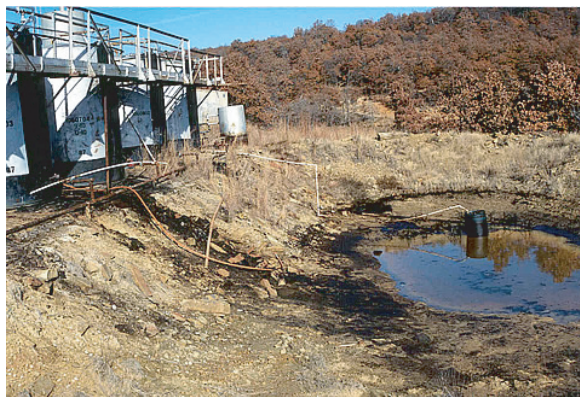
FIGURE 6.1 A tank battery showing produced water discharged to an unlined holding pond in Osage County, Oklahoma. SOURCE: NETL (2006).
